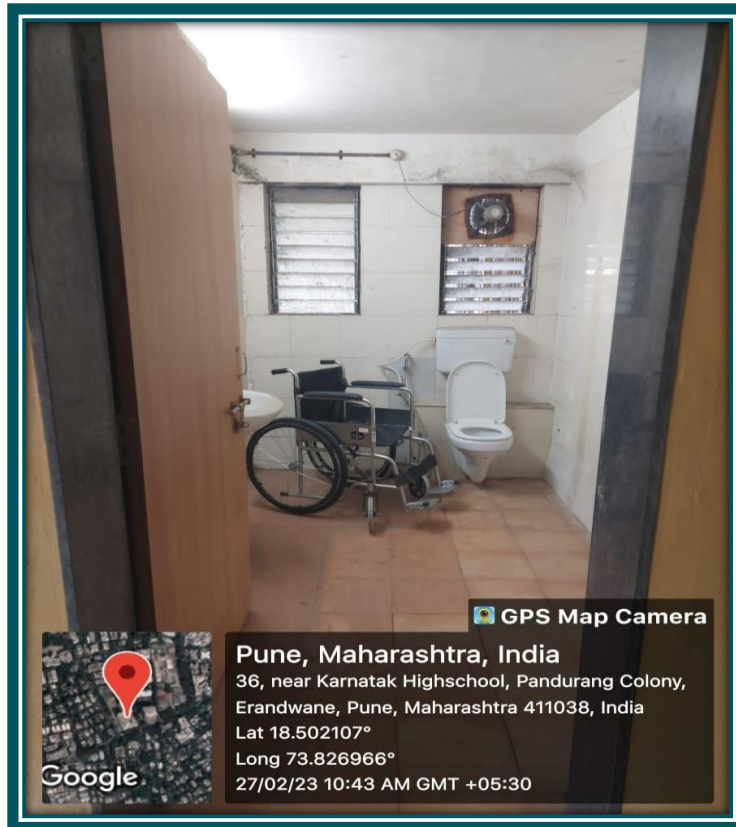
Restroom for Divyangjan on Ground Floor near Ramp
